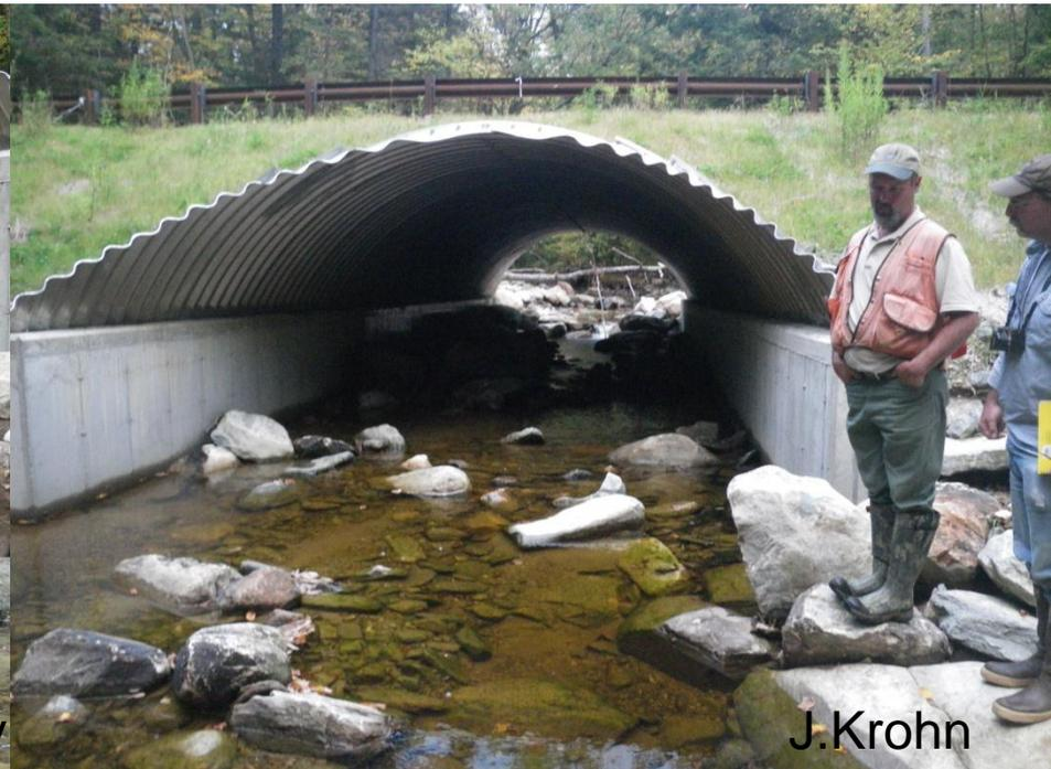
Lost largest boulders near outlet and some roughness along stem walls.
