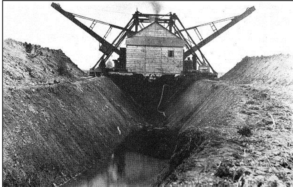
Excavating a large ditch using steam power, circa 1910.
